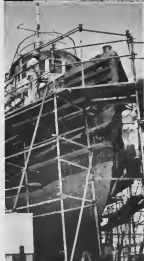
MARINE MANAGER J. H. Brown III and H. GERENTE DI Marina J. H. Brown III y H. H. H. Garje. Floating Equipment division head, Garje, left in division di Floating Equipment, check the propeller shaft (the long one) and its checks e barra di propeller (e soa Largo) y rudder stock. A worker, right photo, checks tronco di timon. Un trahador, porrette na drecha, condition of the tug's smokestack. ta check condicon di e remolcador su chimenea.
